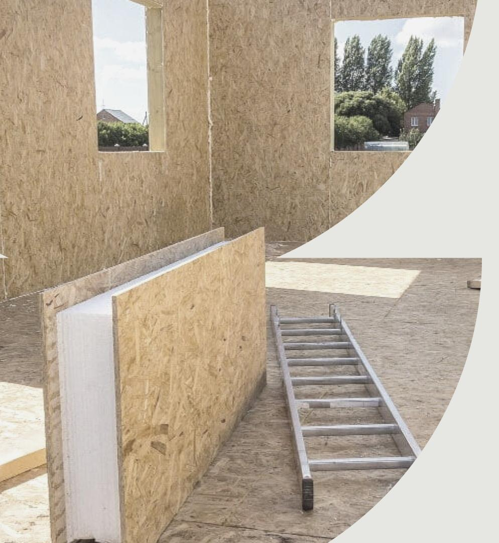
timber-framing methods, total more. Using SIP panels brings the framing time to just 3 days.
