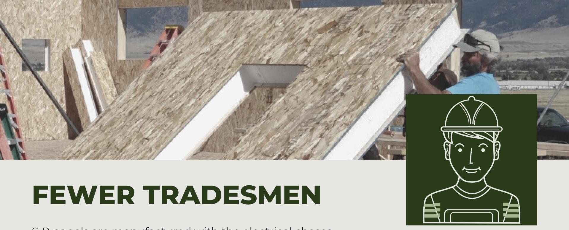
SIP panels are manufactured with the electrical chases already drilled when they are received on-site. The insulation is already there and the exterior is ready for cladding. This all means that fewer tradesmen are needed for construction.
